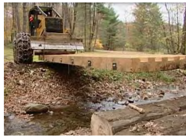
Portable skidder bridge in action, see Figure 16
