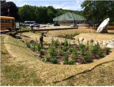
Stormwater treatment in Rutland City, see Figure 22
